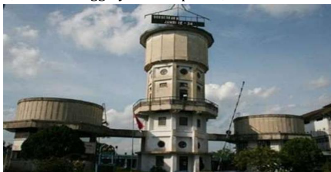
Gambar 1. Menara Air Tua Jambi
