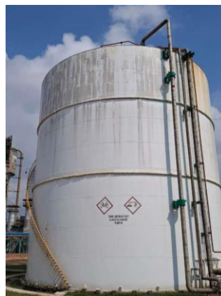
Figure 1. Ammonia Storage Tank 4101-F
