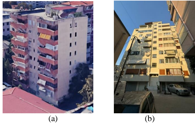
Figure 5. 'Hodo Beg' road, (a) during and (b) after façade renovation
