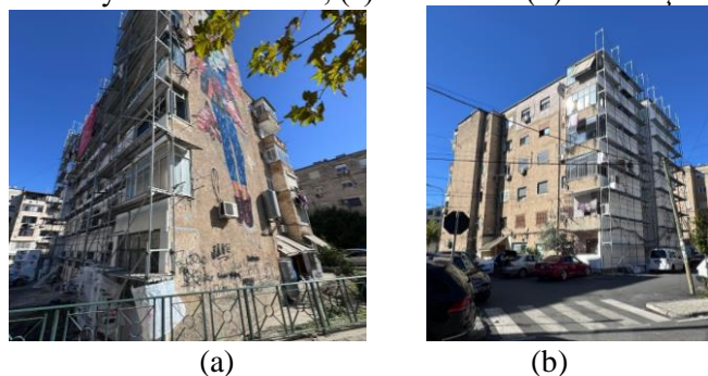
Figure 3. 'Pandeli Çale' road during façade renovation
